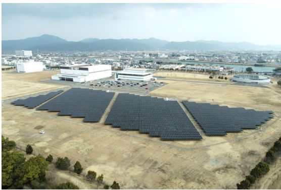
Solar power generation facility at Kitajima Plant
